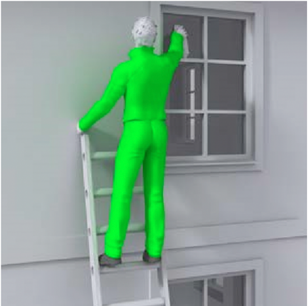
Figure 2 Correct – user maintaining three points of contact (means of securing omitted for clarity)
